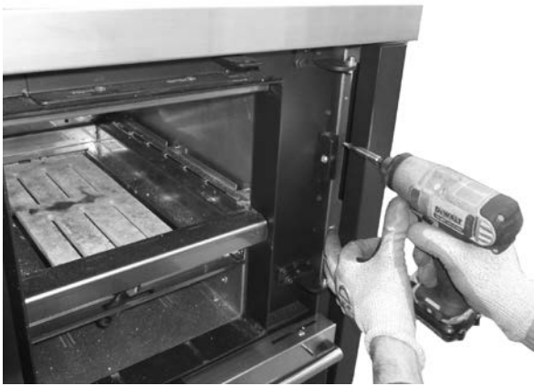
Fig. 27 - Retirer le support
